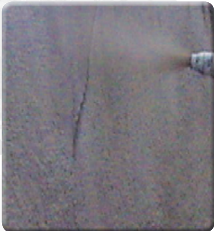
Figure 1. Shotcrete with Microsilica 600 has high build, low rebound and high performance.
