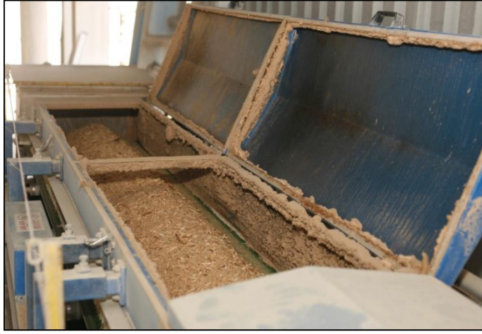
Wood waste feed system inspection hatches.
